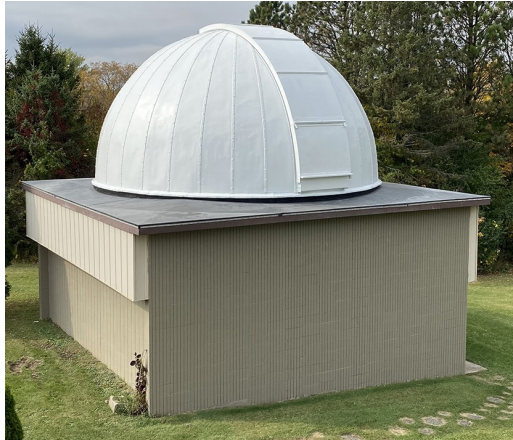
The Z-dome before and after painting
