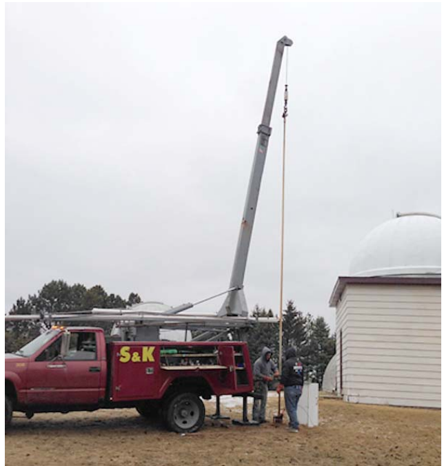
Pulling out the old pump.
