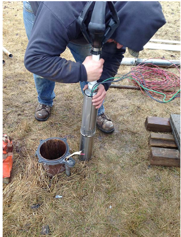
The new pump.
