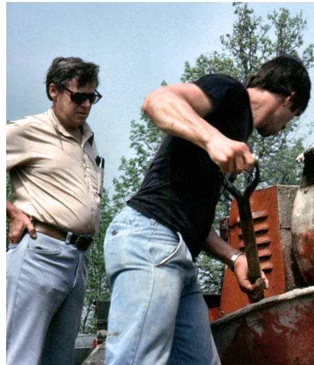
Jim Toeller (left) and Gene Hanson mixing mortar for the construction of the Z building (1980)
