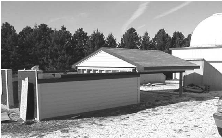
C Scope, Roll-off roof observatory rapidly approaches operational status. Only aluminum cladding the front wall and door hanging remains. Shown at right is the modified Ceola mount on an isolated pad. The mount has a clock drive and is currently being overhauled. Planning is in progress to add digital readouts for RA and Dec.
