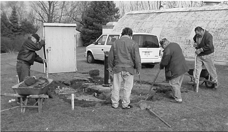
Breaking up the old circular C shed cement Pad
