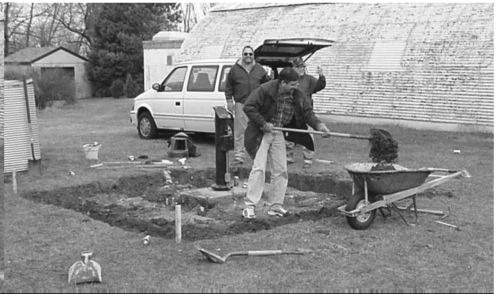
Trenching in the footers for the new 12 x 12 square pad
