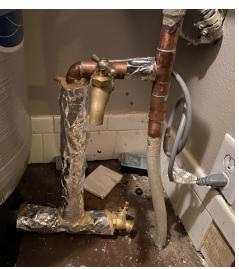
The outlet of the pressure tank (located in the dark room) has been damaged during the last winter and was leaking. We suspect, that even though the room is heated, during some subzero temperature nights the pipe froze. To avoid this from happening in the future Jeff installed a heating tape.
